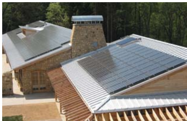
The Aldo Leopold Legacy Center in Fairfield, Wisconsin, features a solar photovoltaic system that produces more power than the facility uses over the course of a year. Homes and businesses across Wisconsin are increasingly turning to solar systems like this for a local source of renewable energy. Credit: Kyocera Solar
