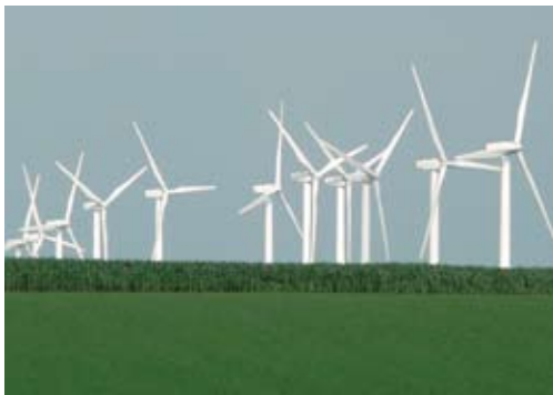
Wisconsin's Blue Sky Green Field Wind Farm began generating electricity in 2008. Credit: Zeke Rice
